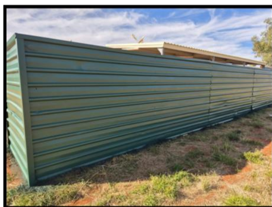
Freshly painted Aged Care fence
