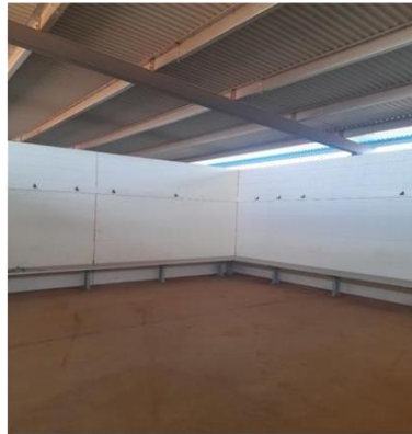
Figure 3. Football oval change rooms.
