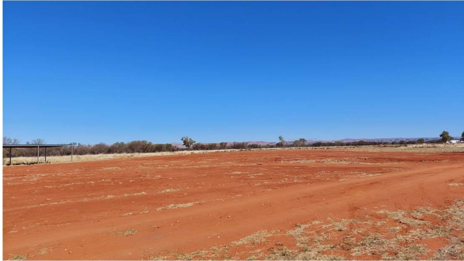
Photos showing clearing of sports grounds
