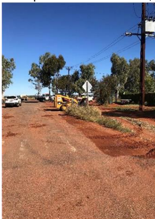
Clearing road verge
