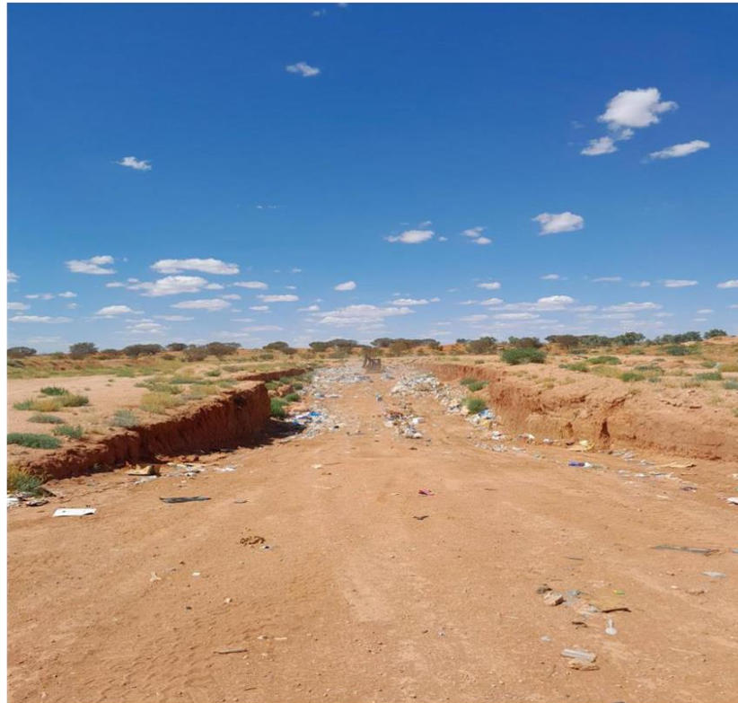
FIGURE 6. Waste pit being pushing.
