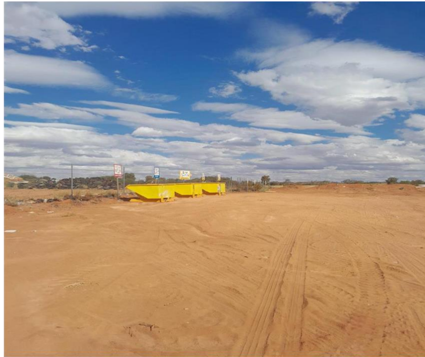
FIGURE 7. Skip bins emptied area cleaned.
