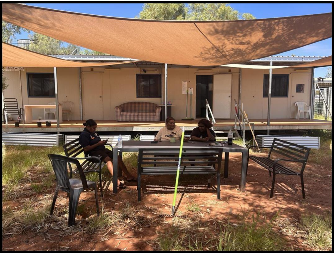
MacSafe team members enjoying the newly completed Yarning Circle
