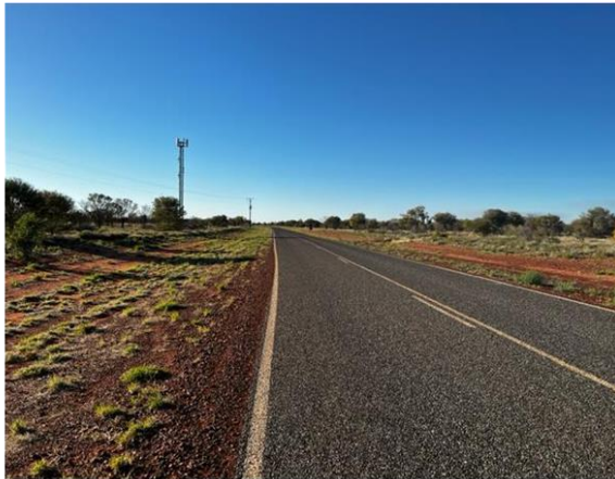
Entrance road looking great thanks to the team
