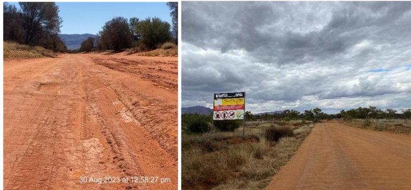
Haasts Bluff internal roads, August 2023
