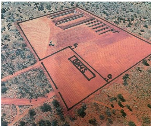
Finke (Aputula) Waste Management Facility
