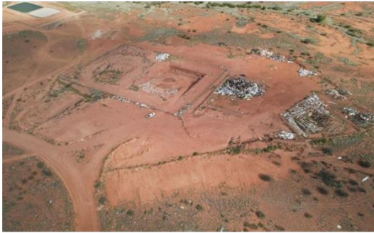
Waste management facility before rehabilitation works
