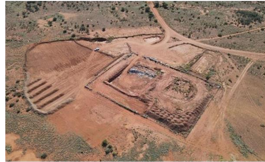
Waste management facility after rehabilitation works
