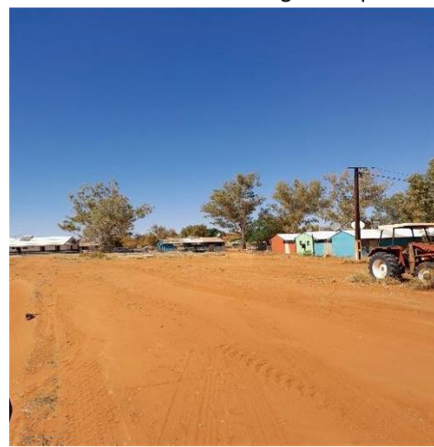
Rubbish & weed clearing from behind houses
