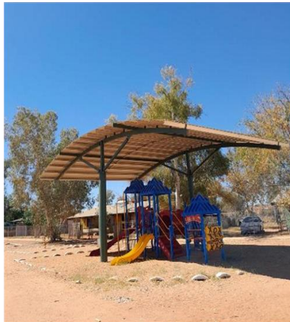
New shade structure at Middle Park
