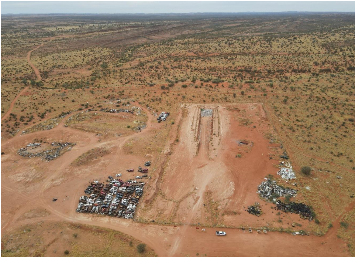
Picture 1: Titjikala Waste Management Facility before remediation
