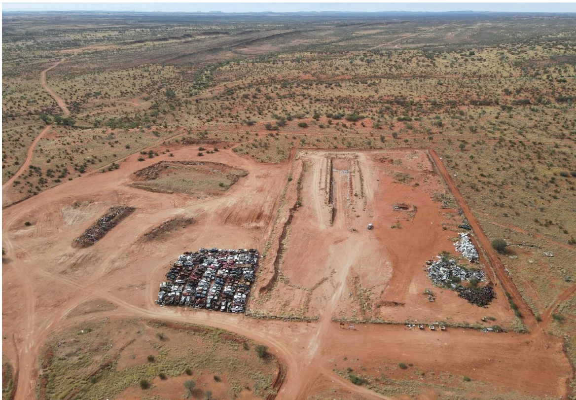
Picture 2: Titjikala Waste Management Facility after remediation
