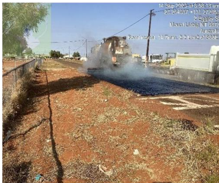
Internal bitumen roads being resurfaced
