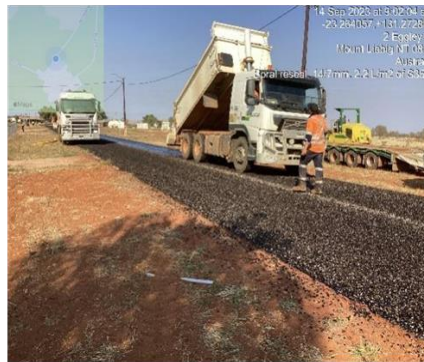
Internal bitumen roads being resurfaced
