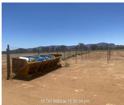
New drop off bays under construction
