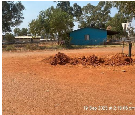
And repairing road shoulders
