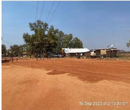
The civil team have been filling pot holes
