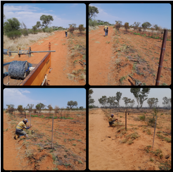
New Boundary Fence
