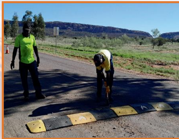
Derek Hayes and Henry Oliver repairing speed hump
