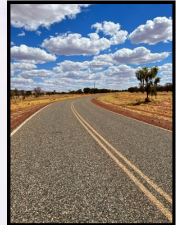
The entrance road edges after being slashed
