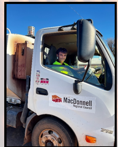
Davin driving the compactor
