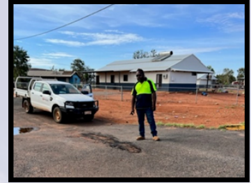
Tristan Road patching
