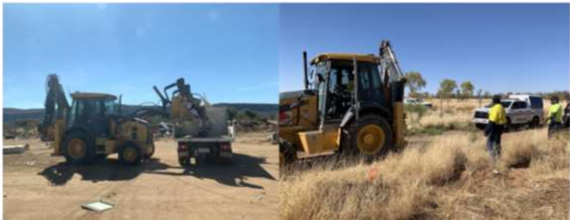
Civil team cleaning up drop off bays
