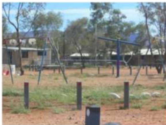
Park requiring some work
