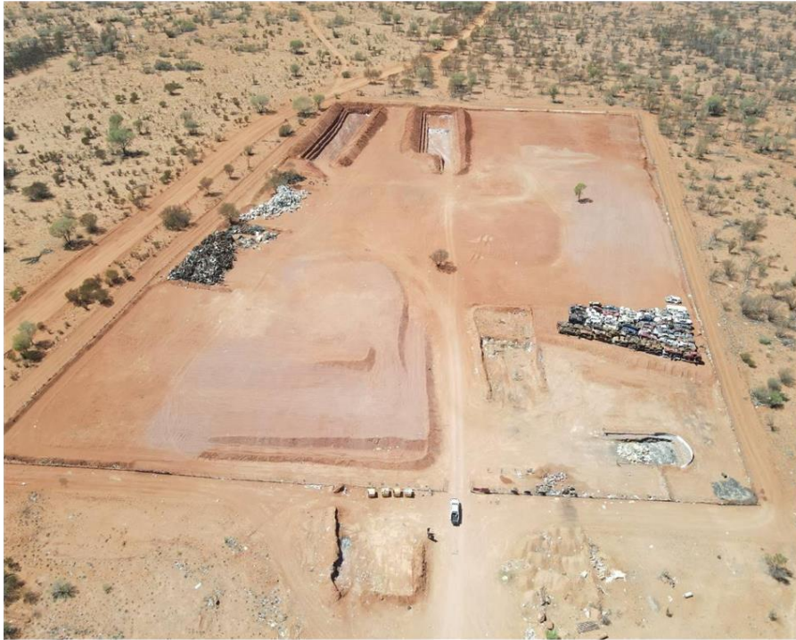
Aerial view of Hermansburg Waste Facility
