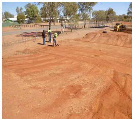
Work at BMX track
