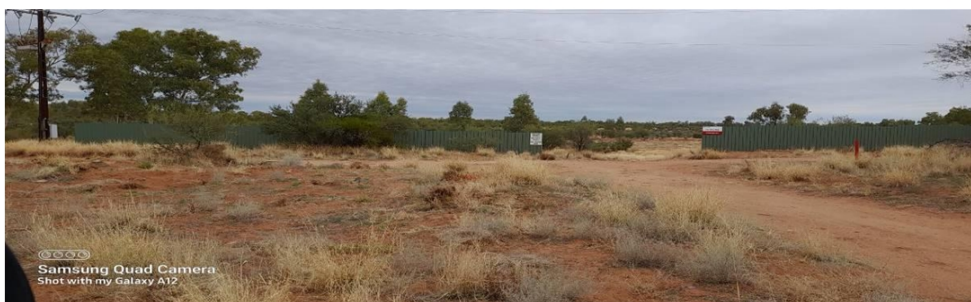
Completed fence with new sign
