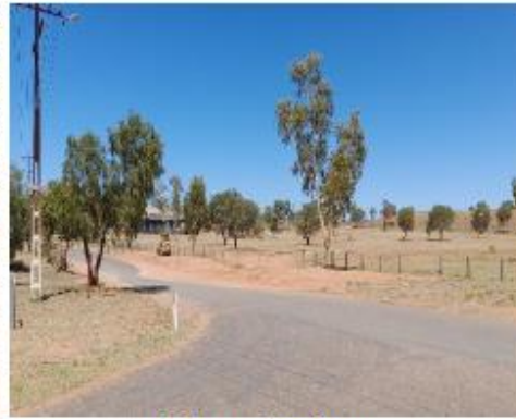
Fixing up floodway
