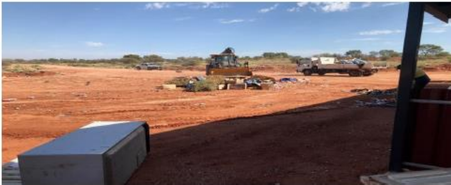
Clean up at the front of separation bays
