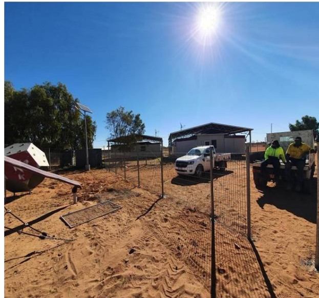
New fence erected at back of park
