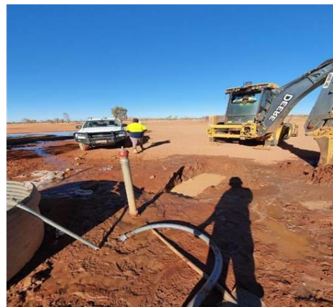
ESO making repairs to town water supply
