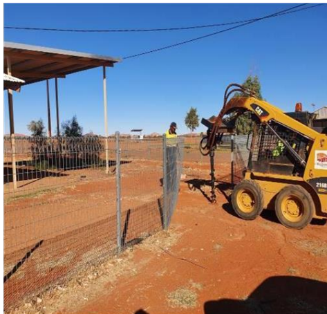
Rec hall fence repairs
