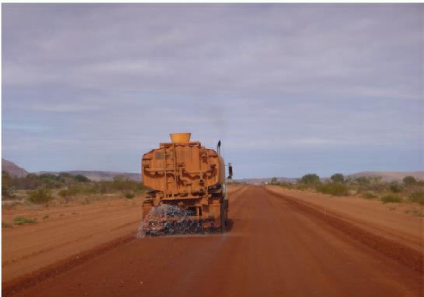
Back-watering after laying out and compacting
