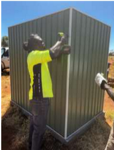
Fig 1: Tristan building the shed at the cemetery
