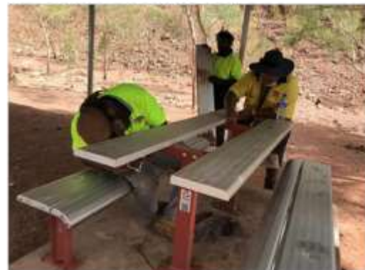
Areyonga Civil Works team repairing table setting
