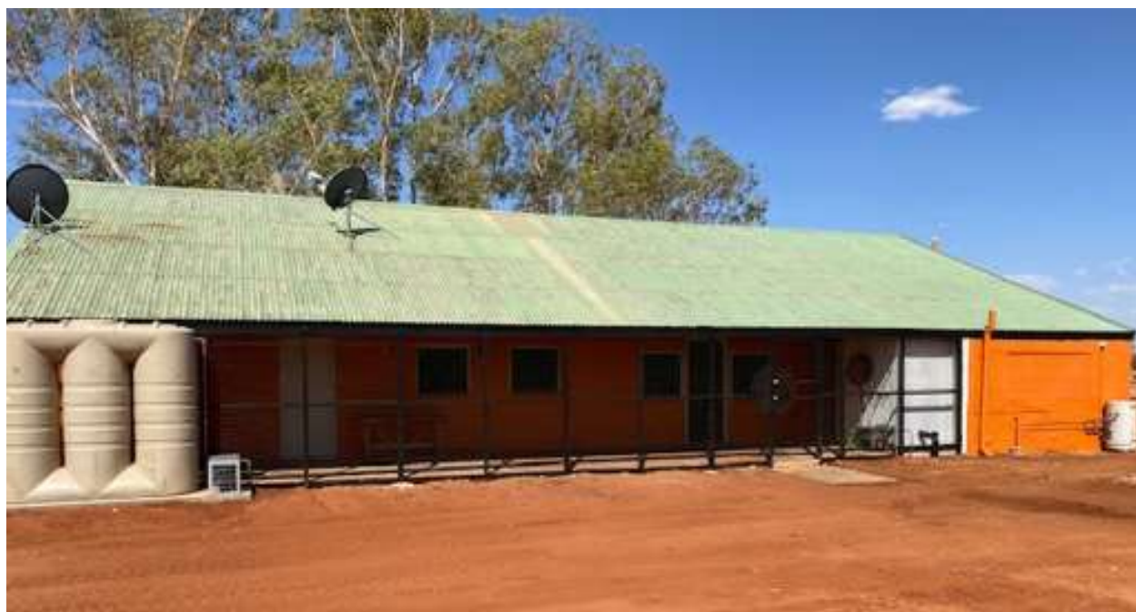
The recently completed Haasts Bluff Aged care facility upgrade funded an Australian Govt grant
