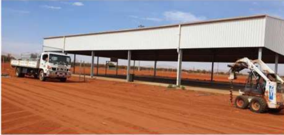
Contractors starting the fence at the Papunya basketball court
