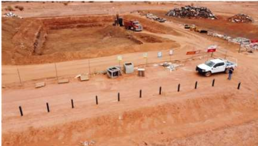
Works progressing at the Imanpa Waste Management Facility
