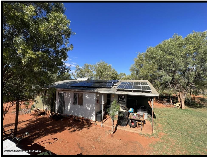
Mount Peachy Solar Inspection
