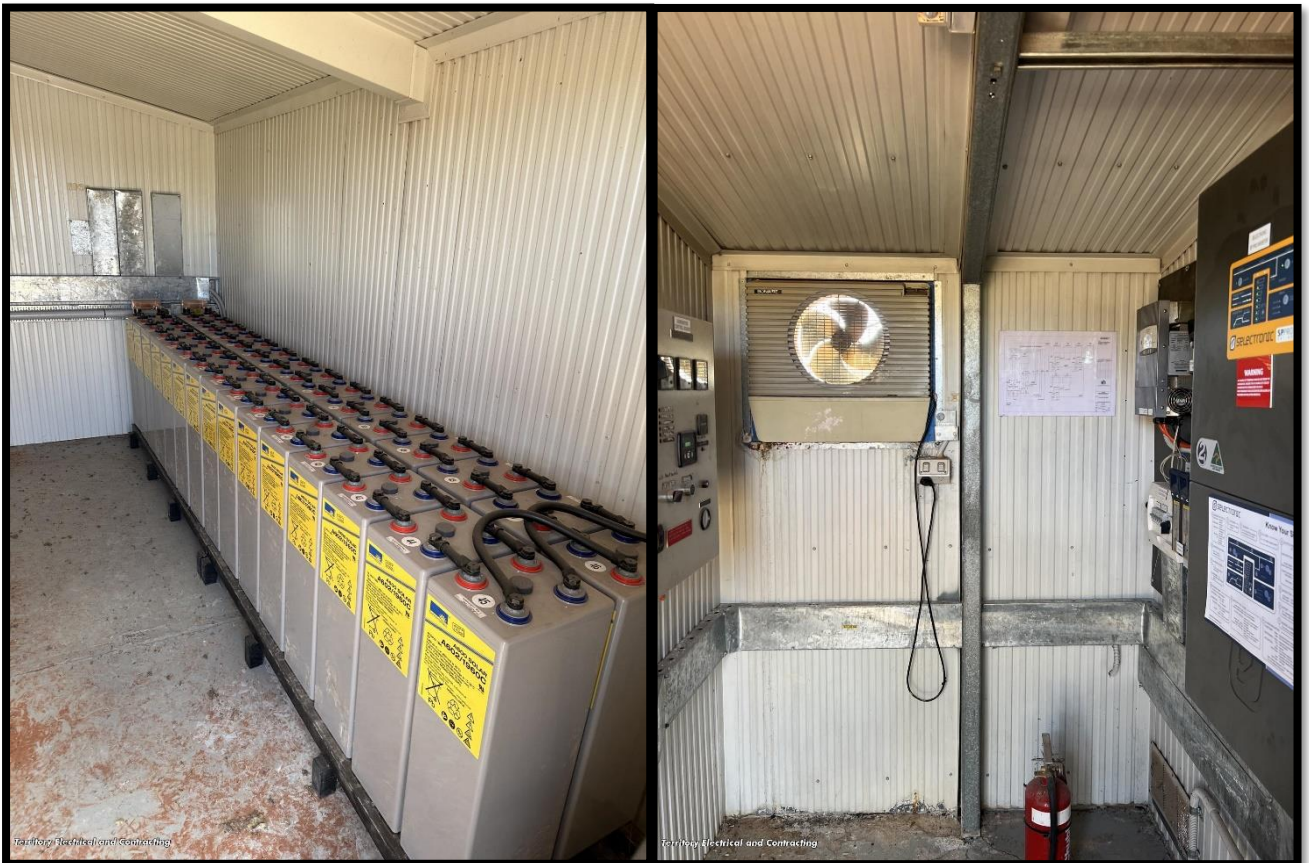
John Holland North and South Solar and Batteries Inspection
