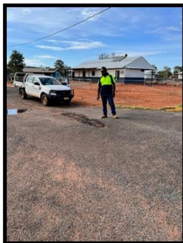
Civil team repairing potholes
