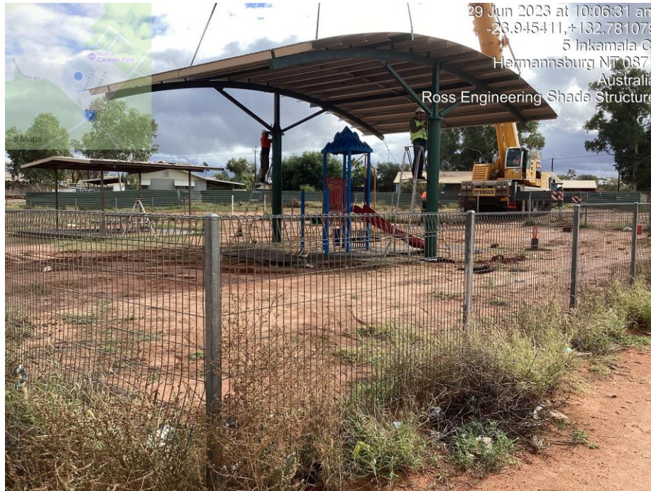
Hermannsburg Shade Shelter craned into place.
