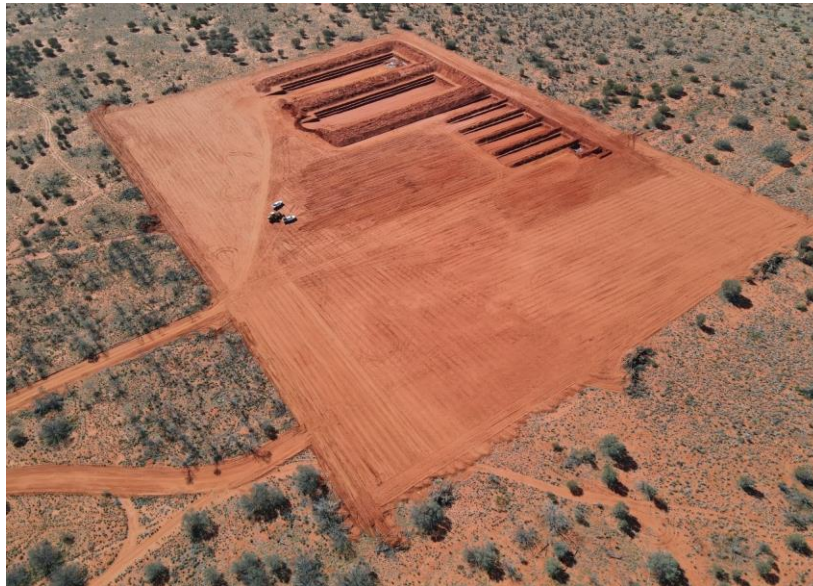
Newly completed Finke Waste Management Facility
