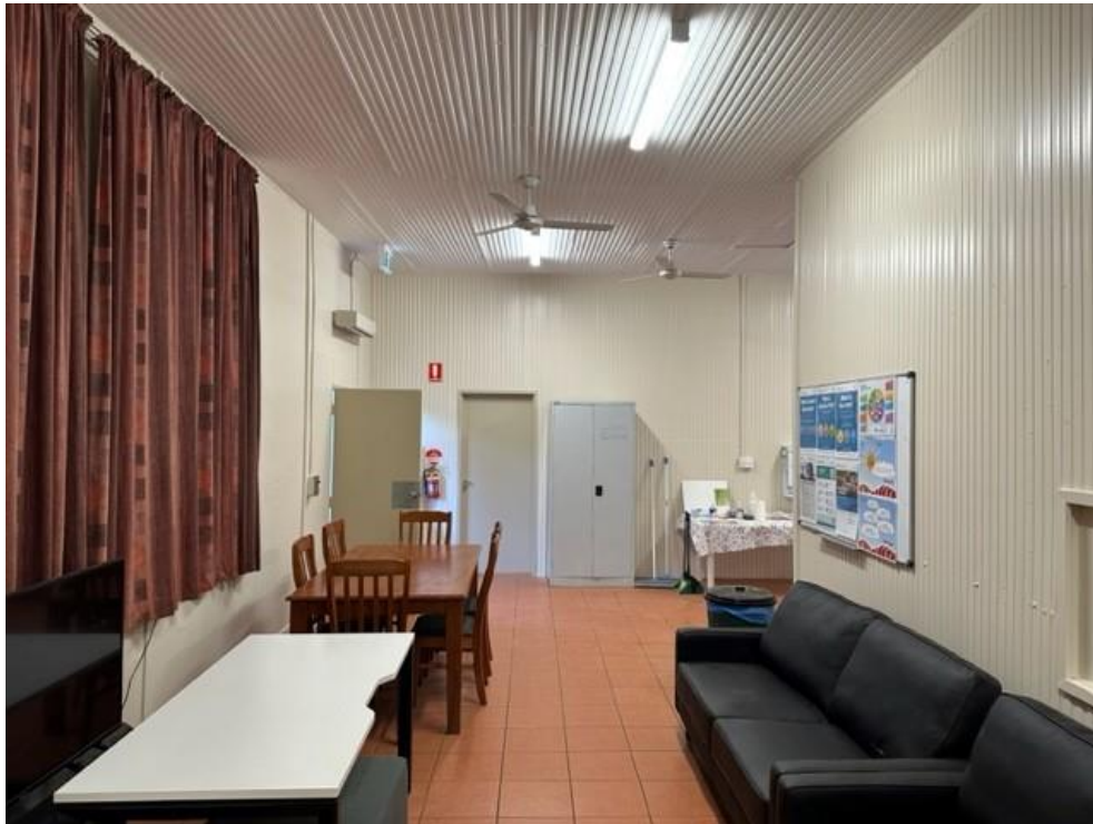
Figure 3 - Areyonga Aged Care internal paint
