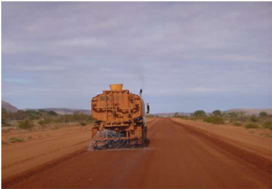
Back-watering after laying out and compacting
