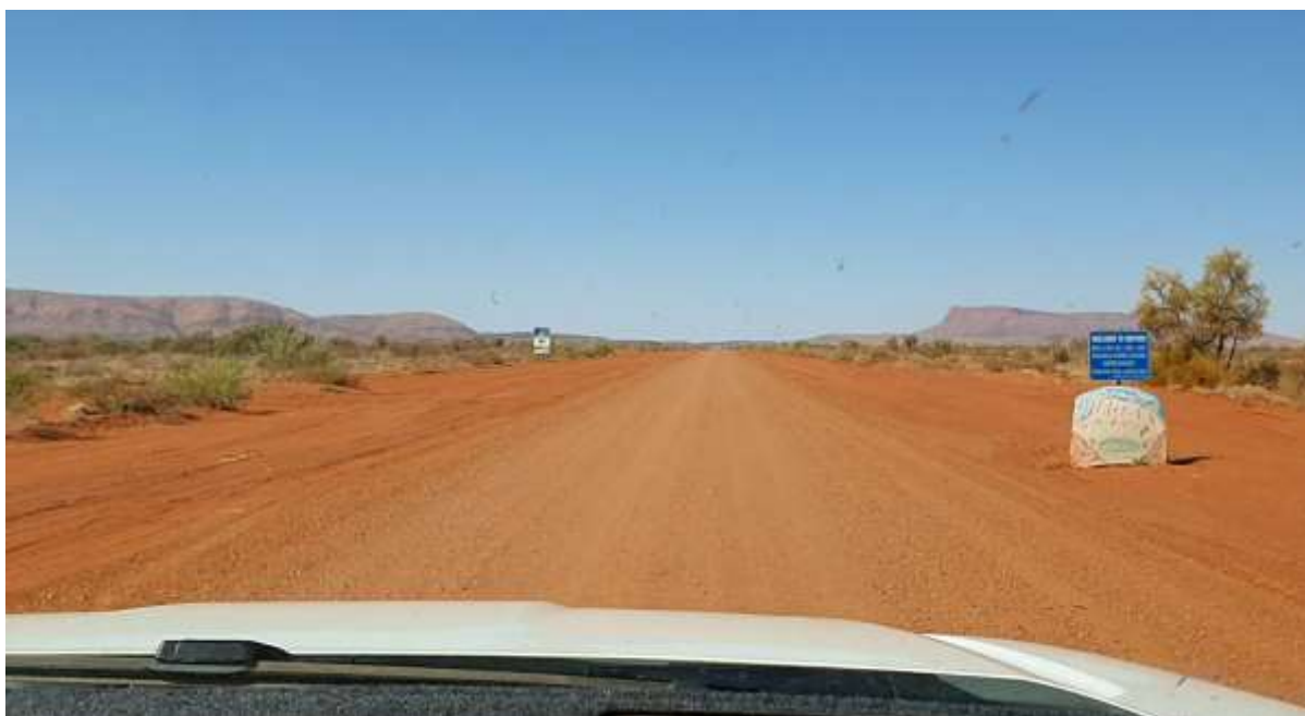
Kintore “highway” nearing completion
