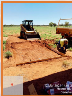
Haasts Bluff civil team laying concrete for the new Cemetery shed
