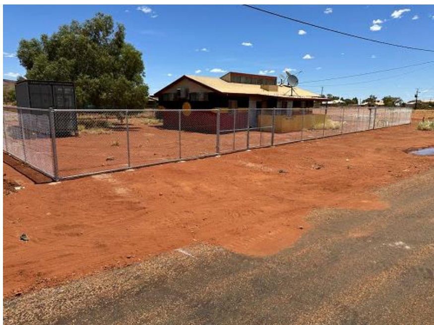
Kintore Drop-in Centre – a fence has been erected around the centre
