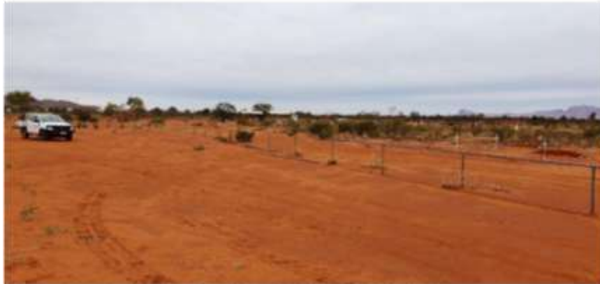
Fence repairs started at Papunya Cemetery
