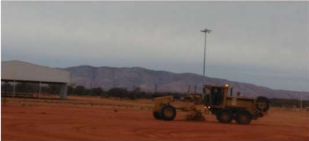
Softball field being graded, Papunya
