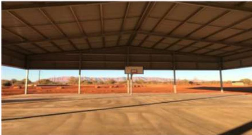
New concrete and hoops for basketball court, Papunya
