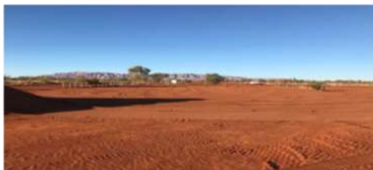
New car park site
