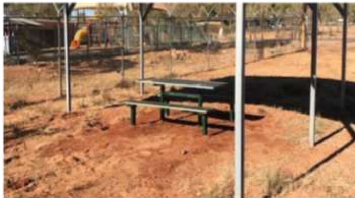
New Seating Installed at pool
