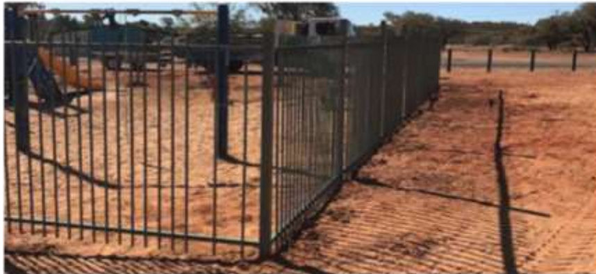
New fence being installed at Eastside Park
