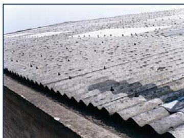
Asbestos Roof Sheets
