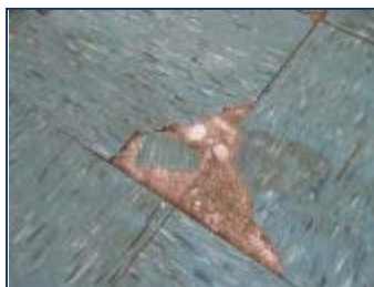
Floor tiles containing asbestos
